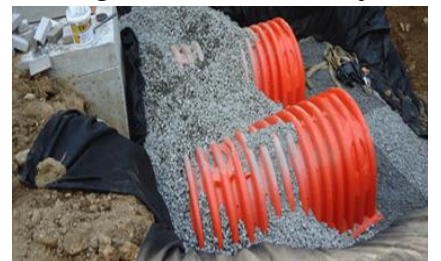
Figure No: 17 Subsurface Detention Systems
