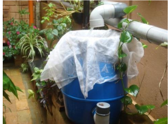
Figure No: 51 Rain Barrel
