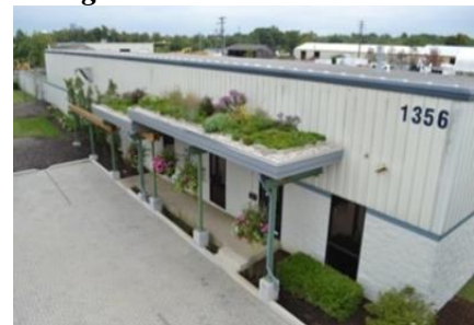
Figure No: 12 Green Roofs
