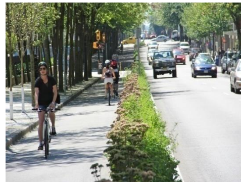
Figure No: 46 Protected Bike Lane Using Planters
