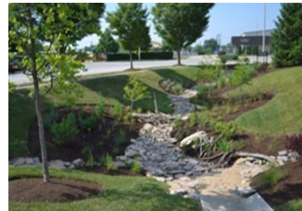
Figure No: 11 Rain Gardens
